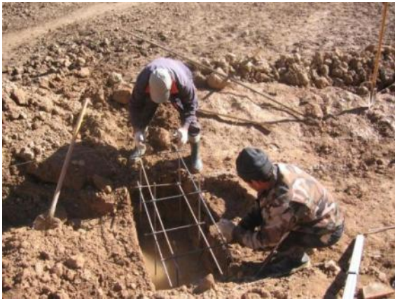
Foundation and Intake
