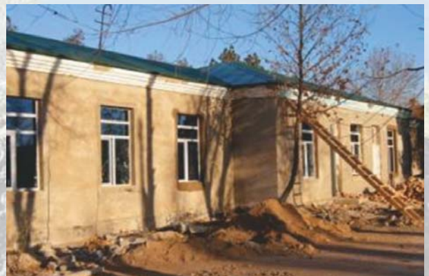
Mastcho Central District Hospital Reconstruction works, 2012
