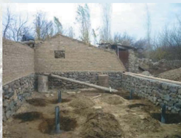
Construction of greenhouses, Konibodom, 2012
