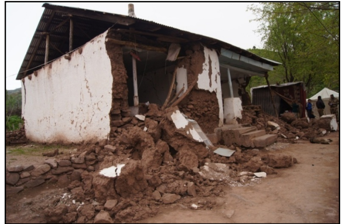
Damaged house in Tavildara district.
