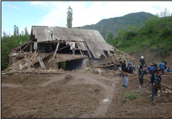
Damaged house in Nurabad district.
